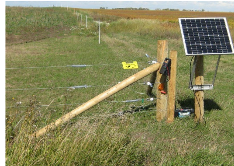
Floating diagonal brace (Source: Kent Solberg | Seven Pines Farm and Fence)
